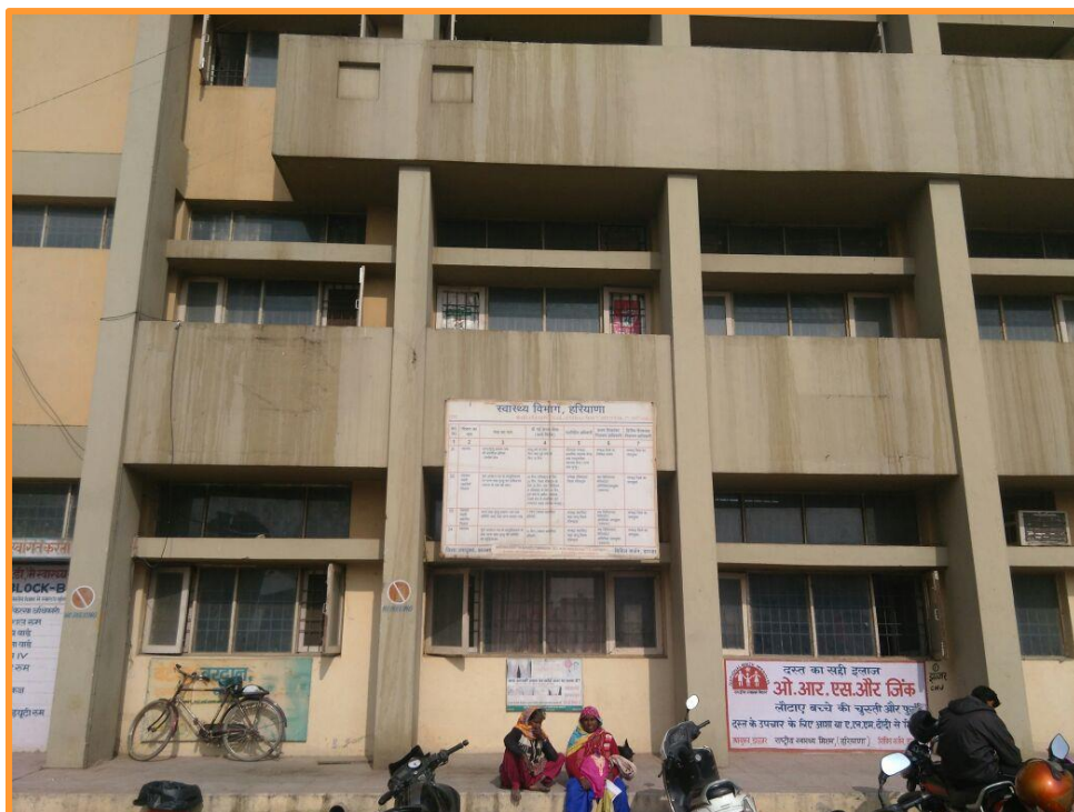
Civil Hospital, Jhajjar
